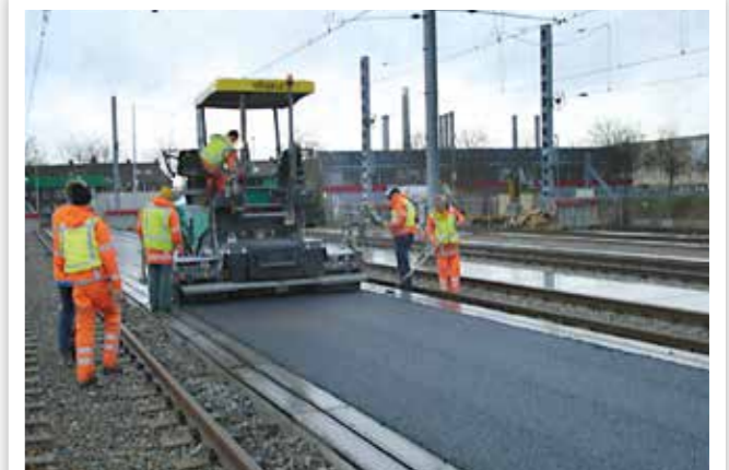
ASPHALT PAVING ON RAILWAY PLATFORMS
