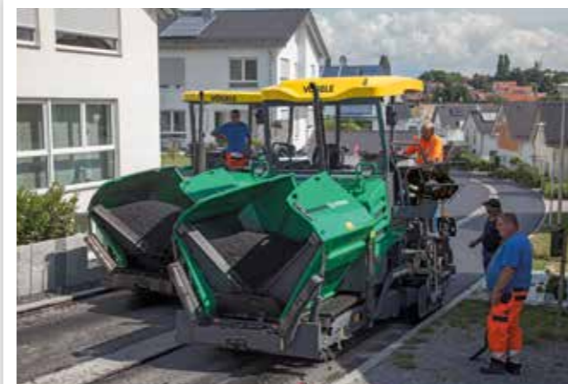
PAVEMENT REHABILITATION ON ACCESS ROADS
