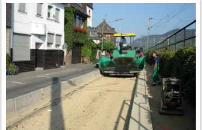
PAVEMENT REHABILITATION ON MUNICIPAL ROADS
