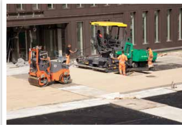
ASPHALT PAVING ON COMMERCIAL SITES
