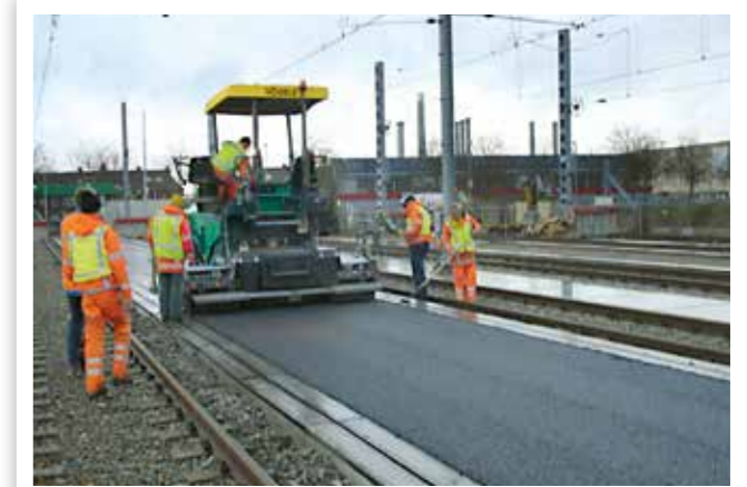
ASPHALT PAVING ON RAILWAY PLATFORMS
