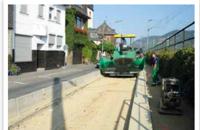
PAVEMENT REHABILITATION ON MUNICIPAL ROADS
