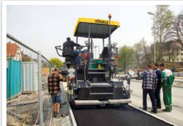
ASPHALT PAVING ON COMBINED FOOT AND CYCLE PATHS
