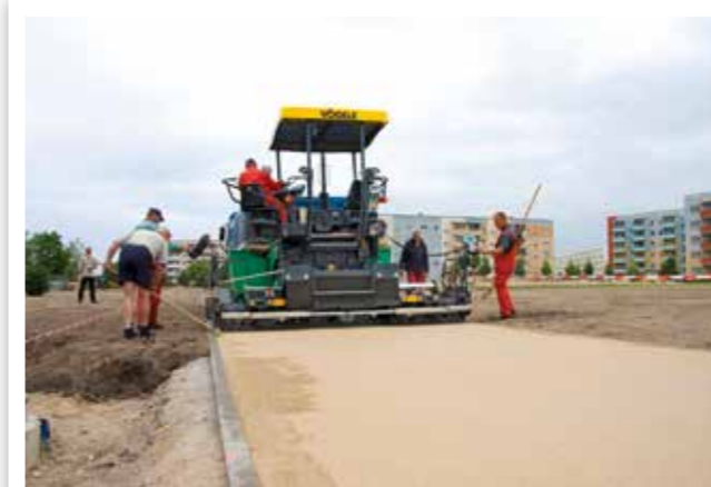
PAVEMENT REHABILITATION ON ACCESS ROADS
