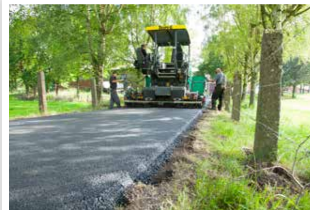
PAVEMENT REHABILITATION ON ACCESS ROADS
