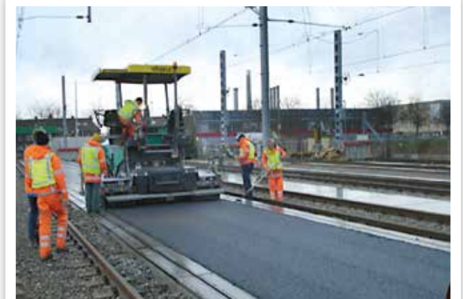
ASPHALT PAVING ON RAILWAY PLATFORMS
