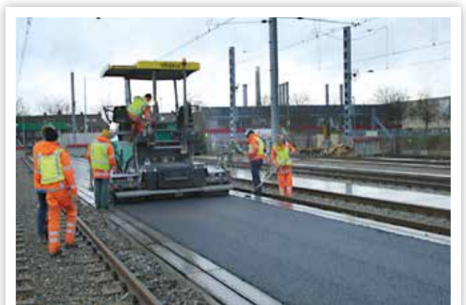
ASPHALT PAVING ON RAILWAY PLATFORMS
