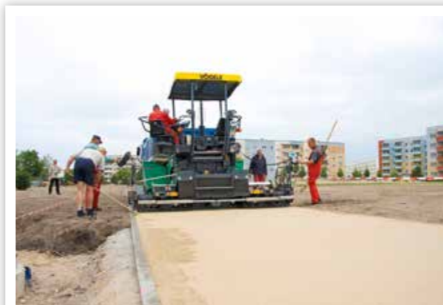
PAVEMENT REHABILITATION ON ACCESS ROADS
