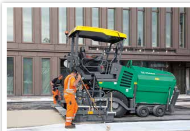
ASPHALT PAVING ON COMMERCIAL SITES
