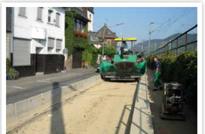
PAVEMENT REHABILITATION ON MUNICIPAL ROADS
