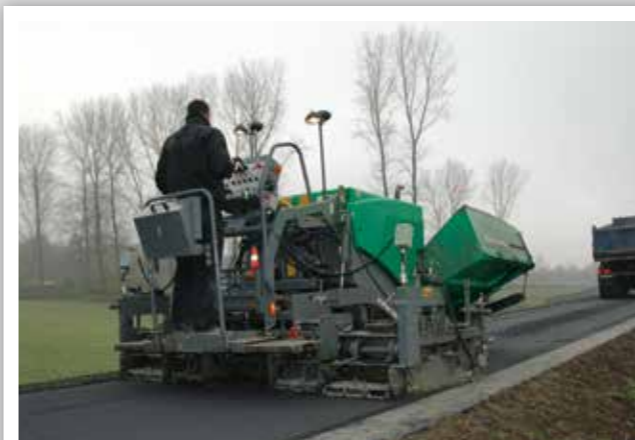
PAVING ASPHALT ON DAMS
