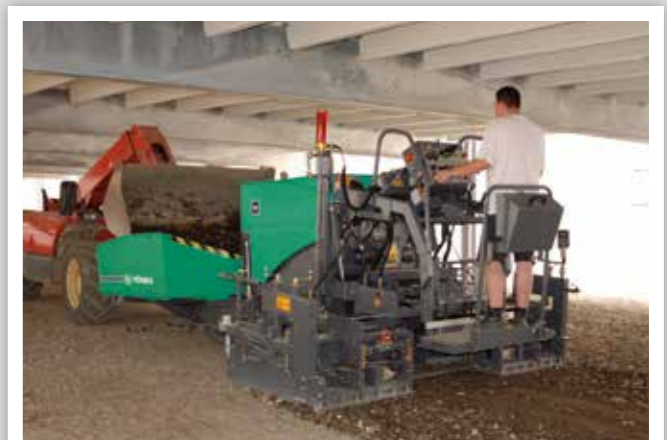
BUILDING THE BASE FOR PAVING SETTS
