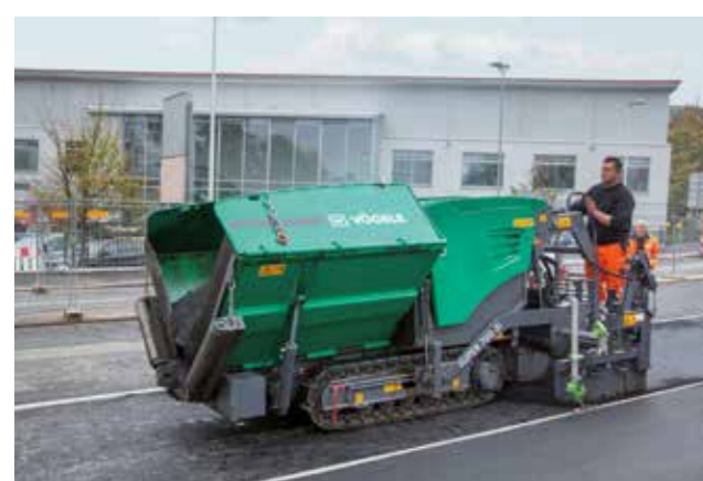
PAVEMENT REHABILITATION ON SMALL MUNICIPAL ROADS
