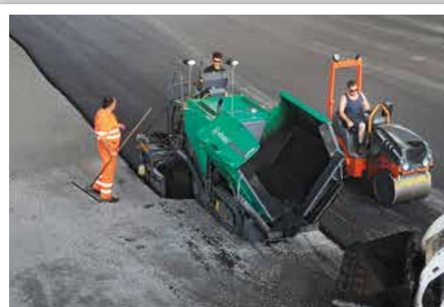
PAVING WORK IN SPORTS FACILITIES
