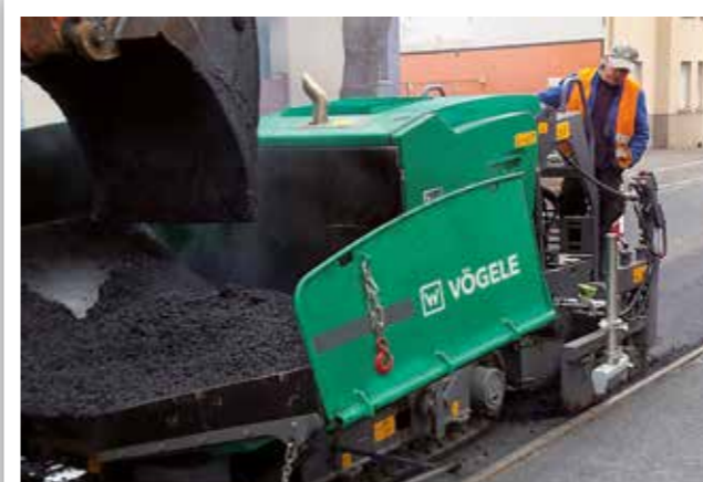
PAVING ASPHALT BETWEEN TRAMWAY TRACKS
