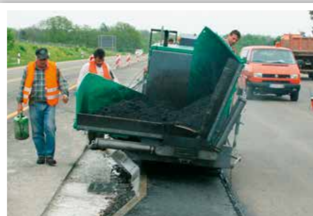
SURFACING MEDIAN STRIPS ON MOTORWAYS
