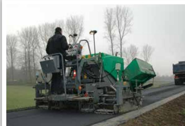
PAVING ASPHALT ON DAMS
