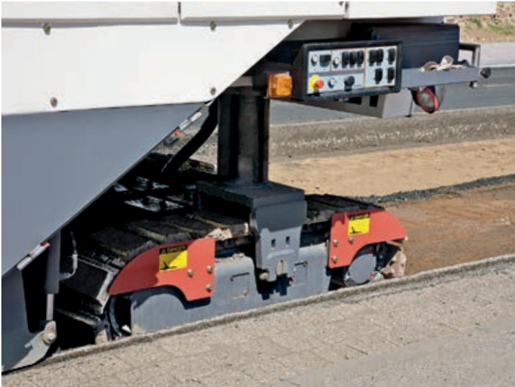
The cold milling machine retains its parallel alignment.
