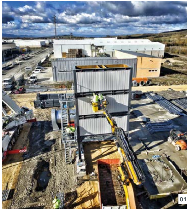
01 Assembly of an ECO plant 02 Disassembly of an ECO plant
