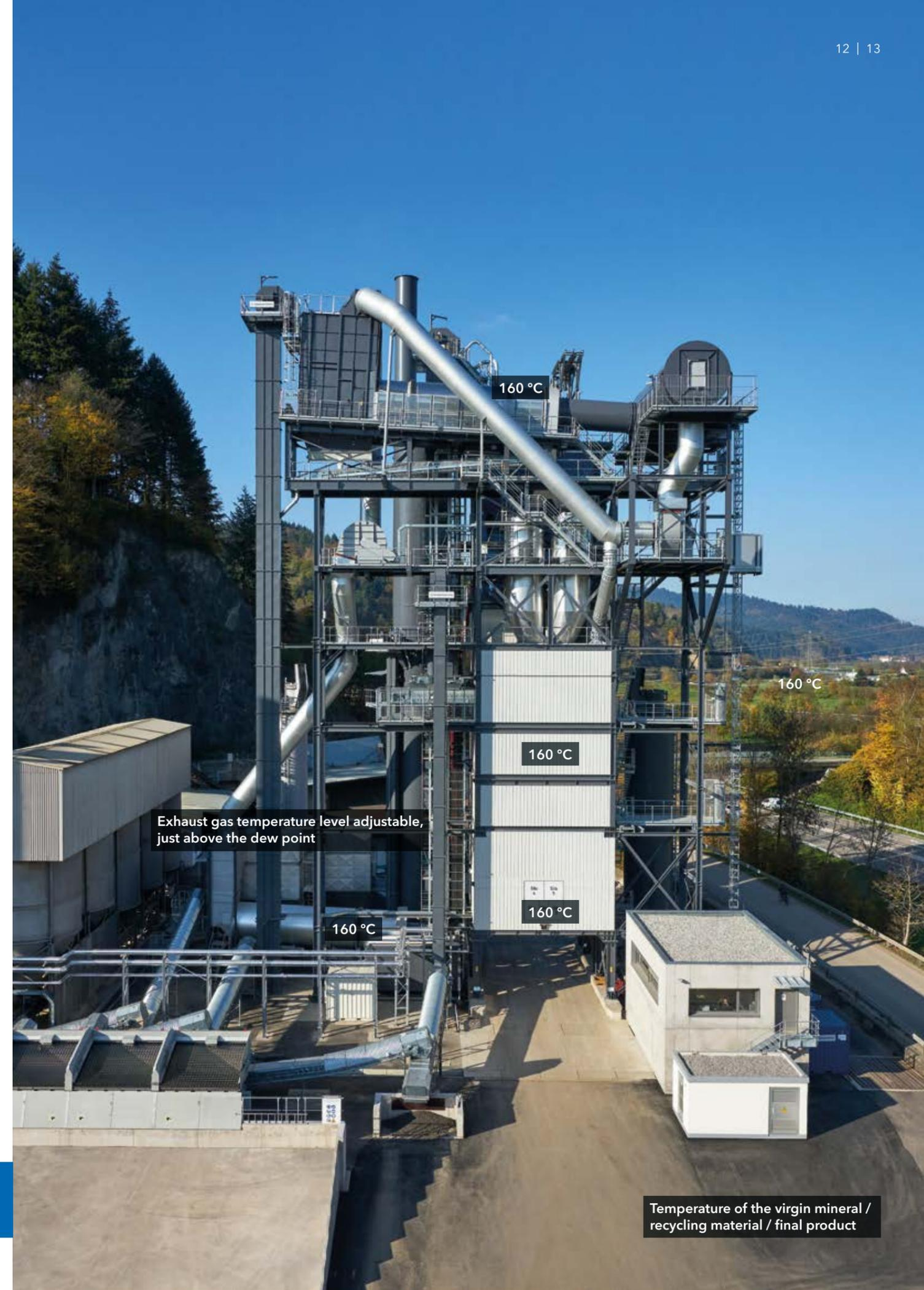
Exhaust gas temperature level adjustable, just above the dew point
