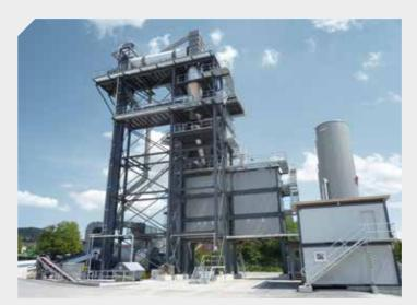
Subsequent expansion of the plant by adding a hot recycling dosing system. With the parallel drum technology, a feed rate of up to 70% can be attained.
