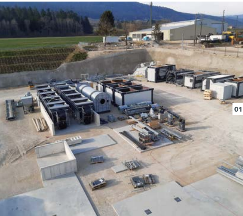
Installation of a TBA plant
