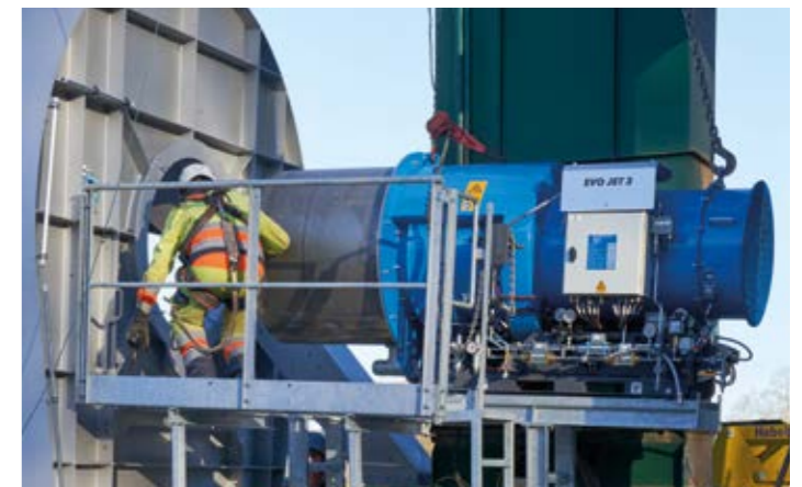
Retrofitting solid fuel burner (wood)
